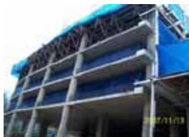
Completed PT Slab
