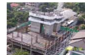
Slip Form Construction with PT Slab under Installation
