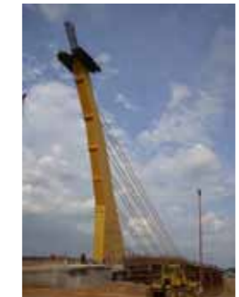
Bridge pylon top for swan head installation
