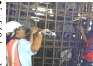
Assembly Dead End Anchorage
