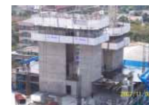
View of Slip Form Core
