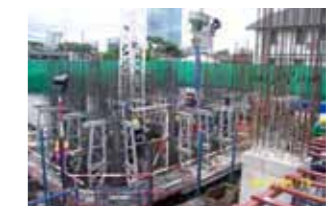
Assembly of Slip Form Equipment
