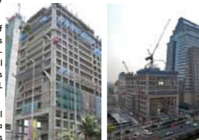
Construction under Progress
