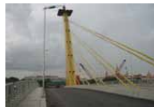
View of completed deck
