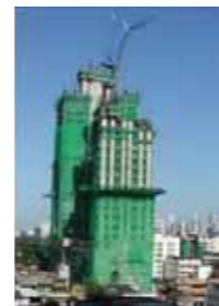
Construction of both tower A & B in progress
