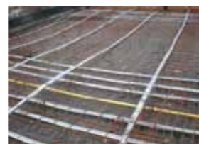
Post tensioning tendons installation ready for inspection prior to concreting
