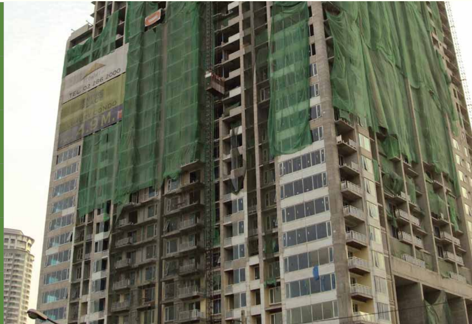
Empire Palace Tower
