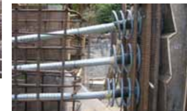
End View of Bridge Girder with Anchorage PBL M 706
