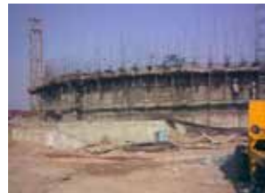
Silo view during slip forming construction
