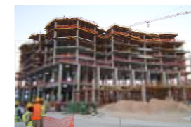
Work progress under construction
