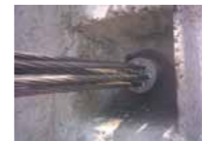
PBL anchorage M705 after stressing
