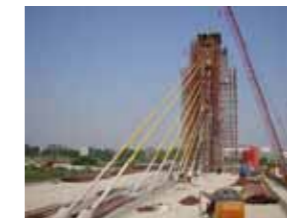
Cable duct installation
