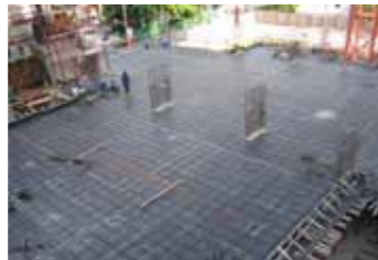
PT Slab of Parking Building
