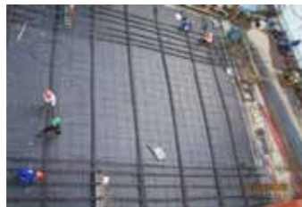
Tendon Layout Parking Slab
