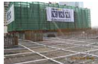
Laying of Post Tensioning Tendons at Sulafa Tower
