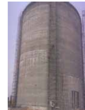
View of silo during final stage of stressing
