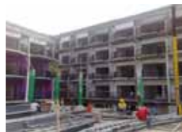
Phuvaree Resort under construction
