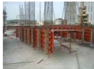
Construction of RC ground floor and columns supporting PT 1st floor at LCC convention building
