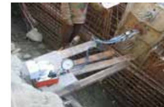
Stressing of Tendon Under Progress
