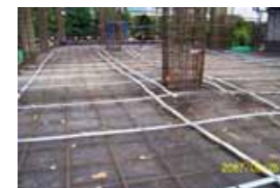
PT Tendons Installation
