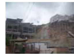
Kamala Falls Resort under construction
