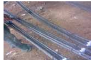
Cleaning of Ground Anchors Free Length
