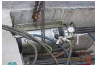
Stressing of Main Transferred Beam at 8th Floor Level
