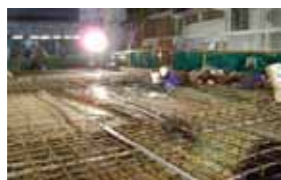
Typical PT tendon for 3 rd floor and other floor
