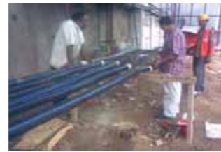
Ground Anchors after Fabrication
