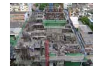
Post tensioning system under construction
