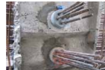
End View of Bridge Girder with Anchorage PBL M 706
