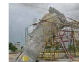
The swan head for installing to the top of the bridge pylon top
