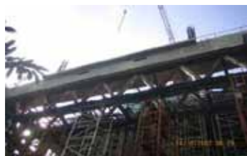
28 m. Span Transferred Beam with Temporary Steel Truss Support
