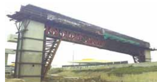
Portal Frame under Construction
