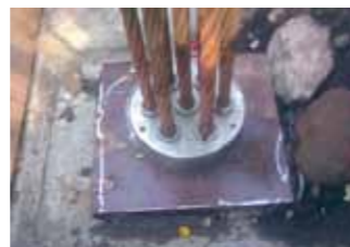
PBL MF706 Anchorage with Trumpet and Bearing Plate
