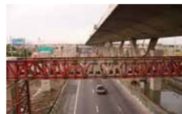
Steel Frame Support the Construction Portal Frame
