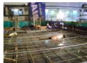
PT tendon under installation at roof floor
