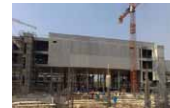
Precast wall was installed into place during construction
